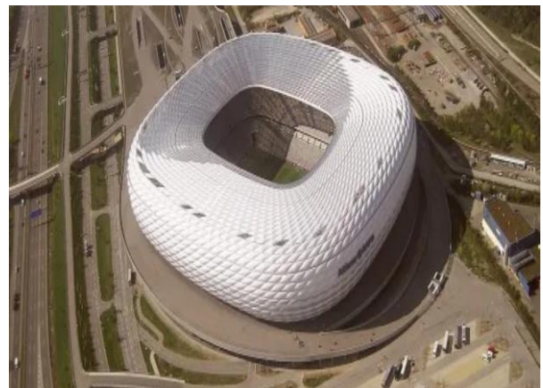
Fig. 22. The Allianz Arena, Munich, Bavaria, Germany, 75,000 Seats, first stadium in the world with a full colour changing exterior. Ref. [24]
