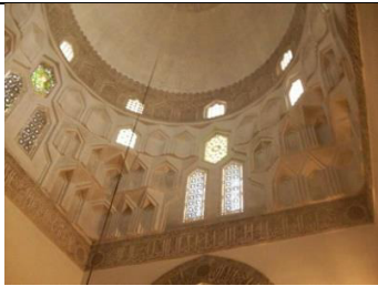
Figure 15 illustrates the dome from inside. Islamic Muqarnas and stained glass were used in the interior design of the Mausoleum dome.
