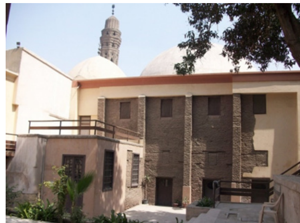
Figure 7 indicates the Entrance of The Dervish Theatre “Sama Khanna-Ottoman Era” which was built on Sunqur Al Saadi school -Mameluks Era. (Photographed by researcher)
