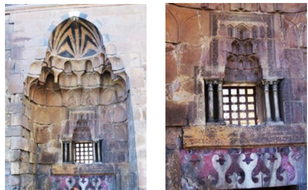
Figure 10 and Figure 11 illustrates a part of the Mameluks gate of Sunqur Al Saadi School. The architectural elements used was “Al Muqarnas” as a Transitional element on the Gate. The Natural Materials used was “Al Ablaq” which is Black and Light Brown Rocks forming the Arch. (By Researcher)
