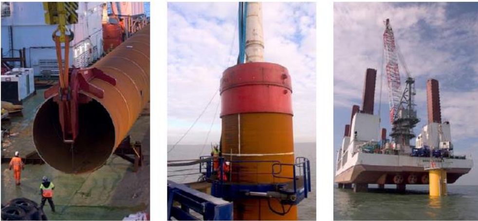
Fig. 1: Installation of the Kentish Flats offshore wind farm. (El-Marassi, 2011)
