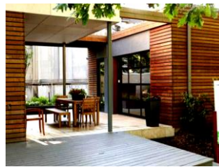
Figure (18): The main entrance
