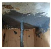
Fig. 5. Surface preparation with epoxy and nails
