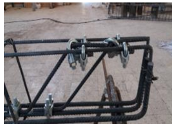
Fig. 1. b.: Bolted tying type.
