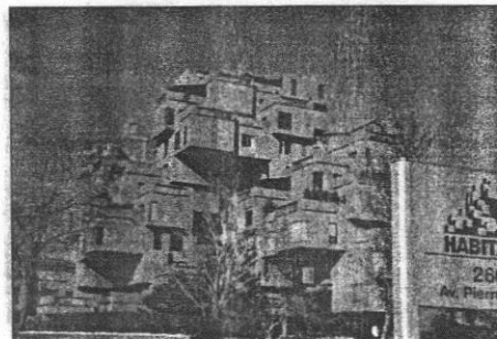
Fig.84, Habitat 67, Montreal, Canada. A residential structure consisting of separate, functional apartments that could be put together in a variety of ways. As people moved in or out, the units could be reconfigured as desired.
