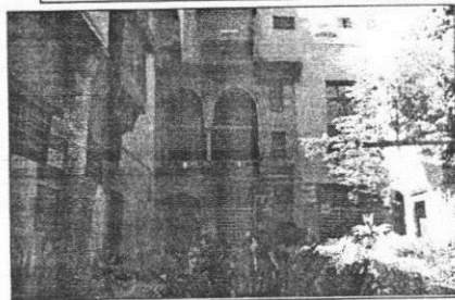
Fig.43, Courtyard balcony (maq'ad) and west courtyard
