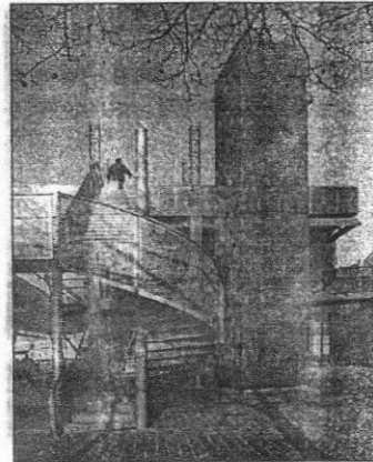
Fig.83, The Parc de la Villette, Paris. The largest discontinuous building in the world.
