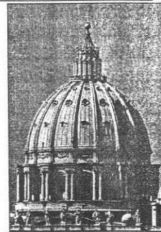
Fig.19, Dome of St. Peter's Basilica in Rome
