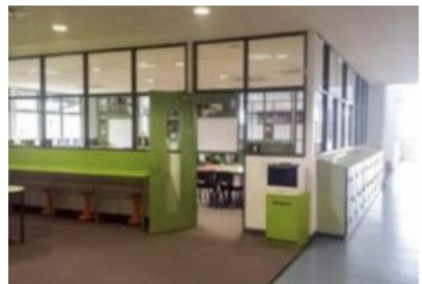
Figure 6: Internal glazing can support a good mix of natural and artificial light
