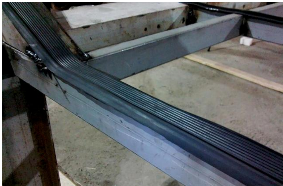
Fig. 4: Lining with vibration-damping material for guides at pipe rolling facility.
