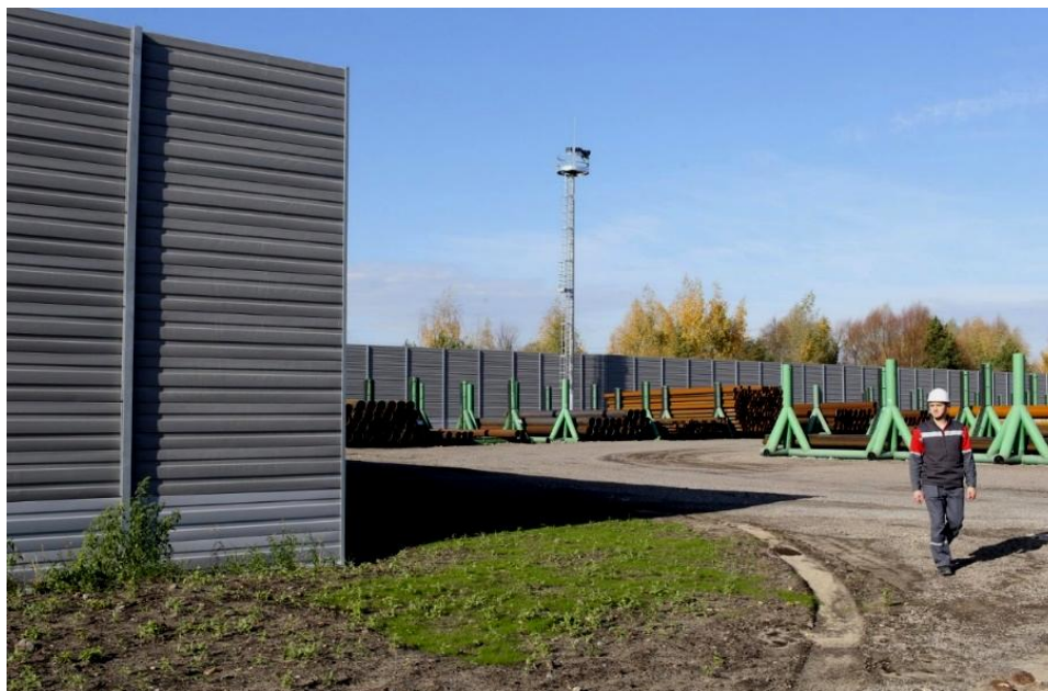
Fig. 6: Noise barrier at Vyksa metallurgical plant along pipe electric welding shop.
