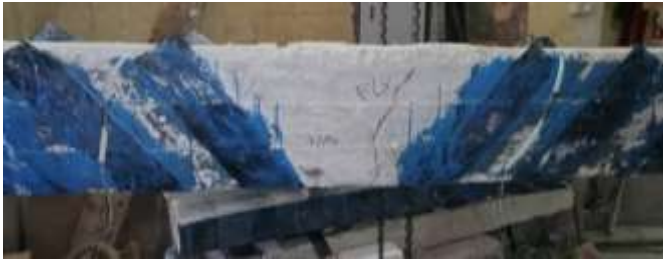
Figure 10: Tested RC beams (B5-II-15) flexural failure
