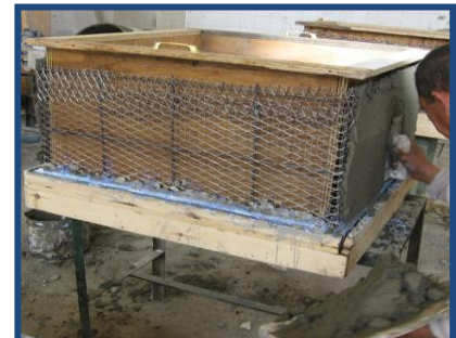
c) Tank walls
