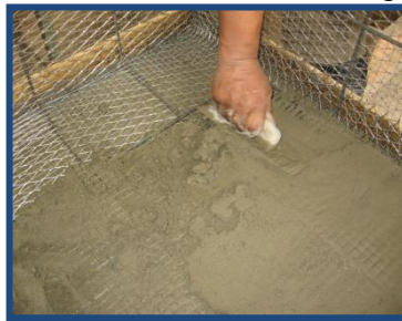
b) Casting the second layer of the base mortar
