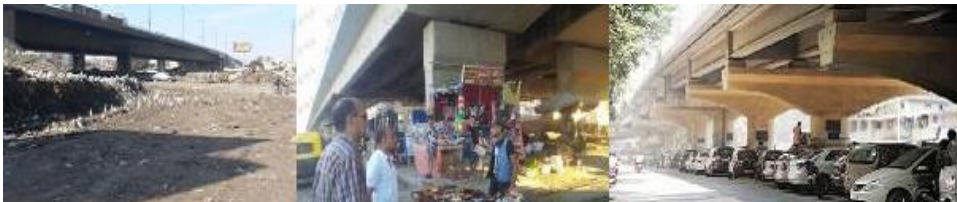
Figure 2 The current situation below the upper bridges in Egypt
