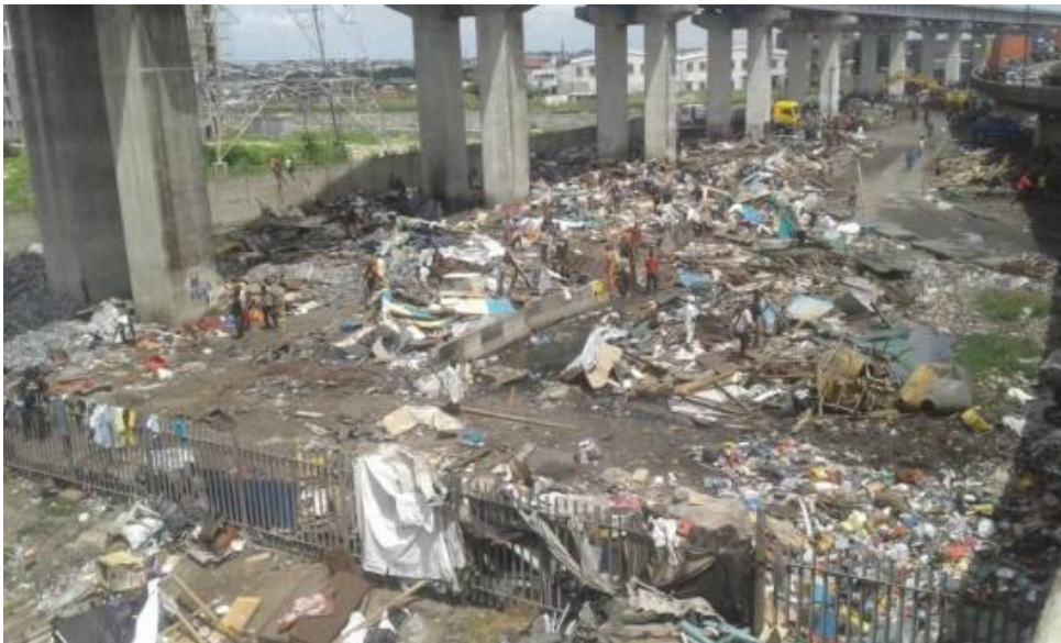
Figure 1 Unused spaces under the upper bridges
