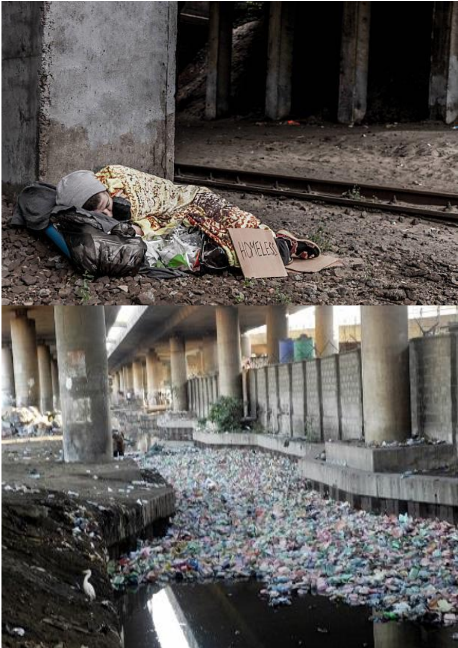
Figure 1 Unused spaces under the upper bridges
