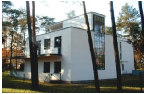
Fig. (5): Walter Gropius' house in Dessau, where the use of white color, straight lines and simple materials with glass.
