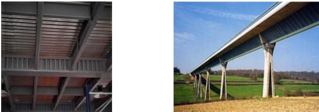
Fig. 1. Usage of GCWs in buildings and bridges
