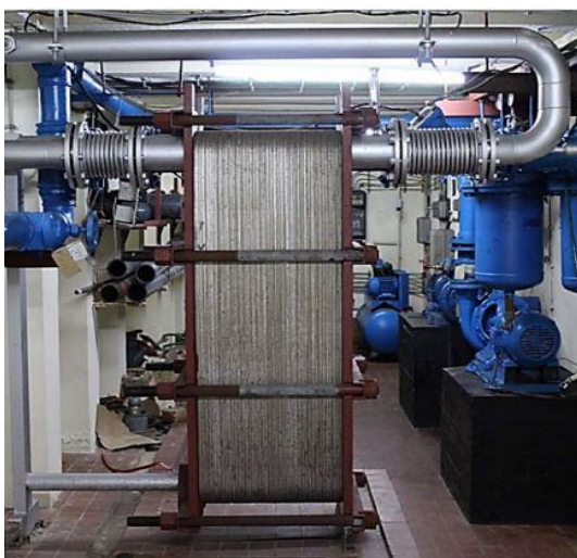
Fig. (4): Heat exchange (left) and Pumps (right) of the primary circuit. [picture took by H. Beya]
