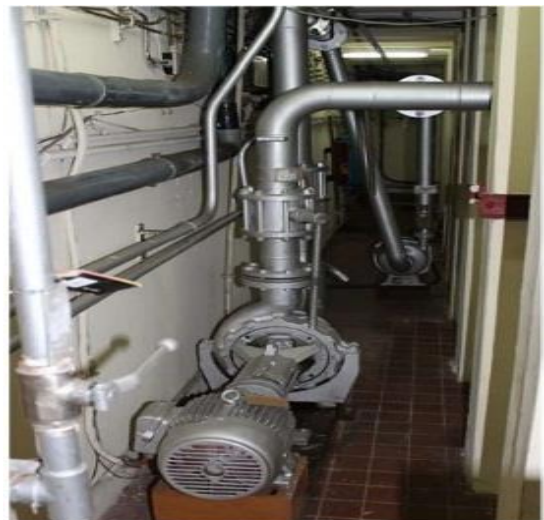
Fig. (4): Heat exchange (left) and Pumps (right) of the primary circuit. [picture took by H. Beya]
