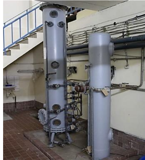
Fig. (2): Ion-exchange and activated carbon filter [picture took by Beya]
