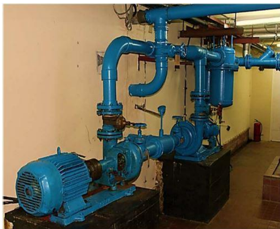
Fig. (5): Pumps and filters (left) [picture took by H. Beya] and cooling towers (right) [picture took by S. Ilunga] of the secondary circuit
