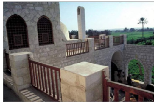
Roof and Balconies View.
