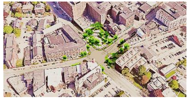
Figure 9: Current Site View for Congress Square Plaza, Portland, Maine [16, p. 7].
