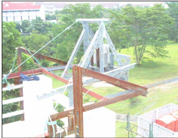
Fig. 3 Rig positioned on top of tower
