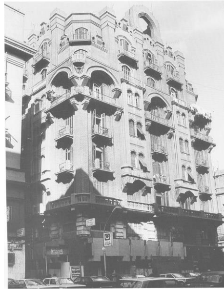
Fig 3: The main façade of the building from Kasr Elnil Street
