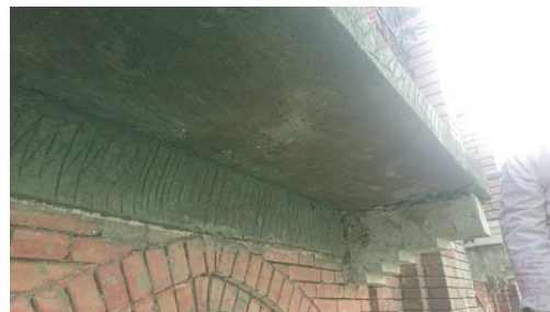
Figures 10: Restoration of Balconies floor concrete
