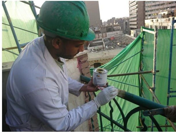
Fig 13: removing over paintings from metal handrail
