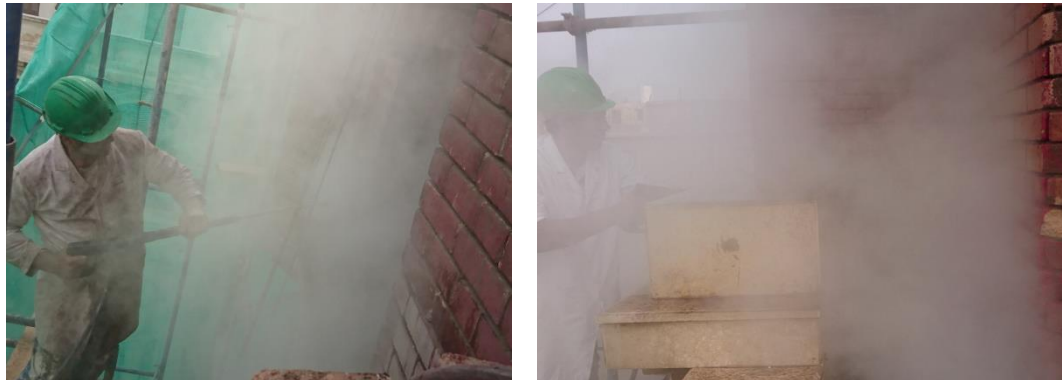
Figures 8: Cleaning the facades with steam cleaning system
