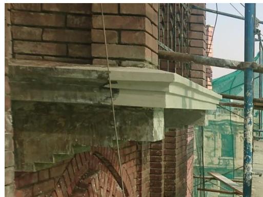
Fig 12: integration of missing parts
