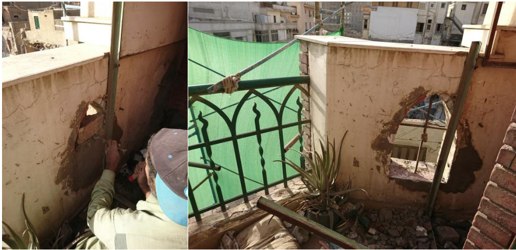
Figures 7: Reopening of the closed old openings
