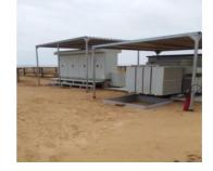
Photo.5. Inverters and transformer
