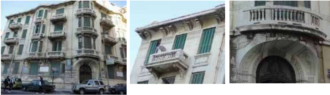
Fig. 10 : Ornamental details of an Eclectic Style residential building façade; the main entrance at the corner with classic panels and decorative foliage, balcony balustrades of repetitive ionic columns, brackets with volutes supporting balconies, a frieze surrounding the top of the building and another at the middle with a bas relief geometric pattern. (Azaritah District)
