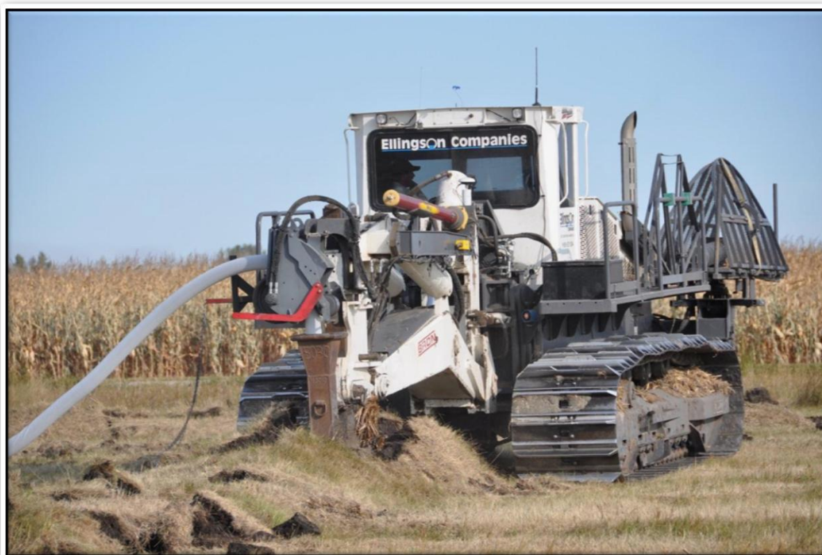
Fig. 12b. Large modern agricultural equipment can create severe compaction and related problems in soil, such as during installation of drain tile near Fargo, North Dakota, USA. Photo by Brevik
