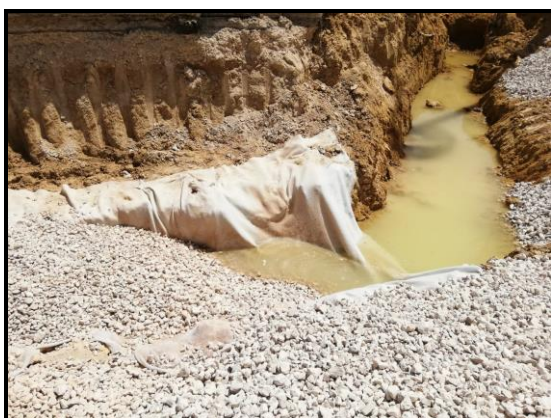
Figure 16. Side open ditch (trench)
