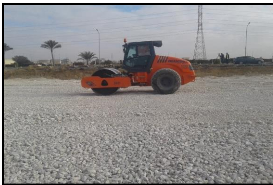
Figure 12. Show compaction of filter layer above rock fill
