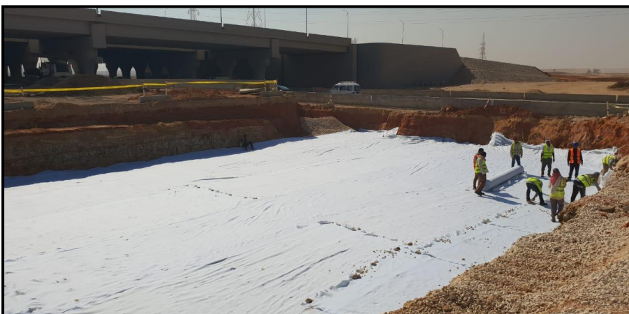
Figure 12. Show compaction of filter layer above rock fill
