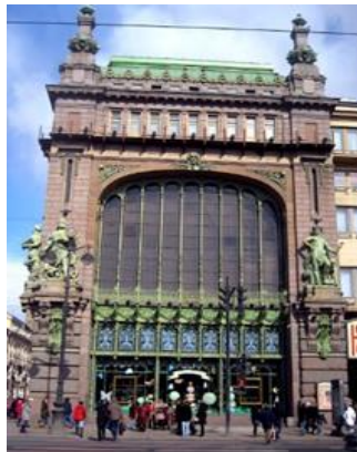
Fig (1) Eliseyev Emporium (1903) in ST. Petersburg, Russia Source: History of Architecture
