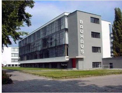
fig (2)– Bao House School Source: History of Architecture
