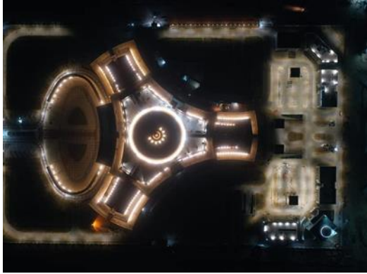
Fig (13) layout -Parliament building in the new administrative capital Available on: https://www.arabcont.com/english/project-589 last Access 27-5-2022
