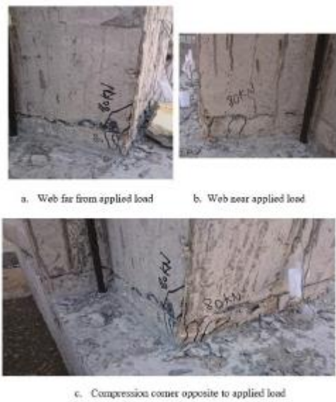
Fig. 11 Crack pattern of specimen (S1s-0.5Pys-0.05P)
