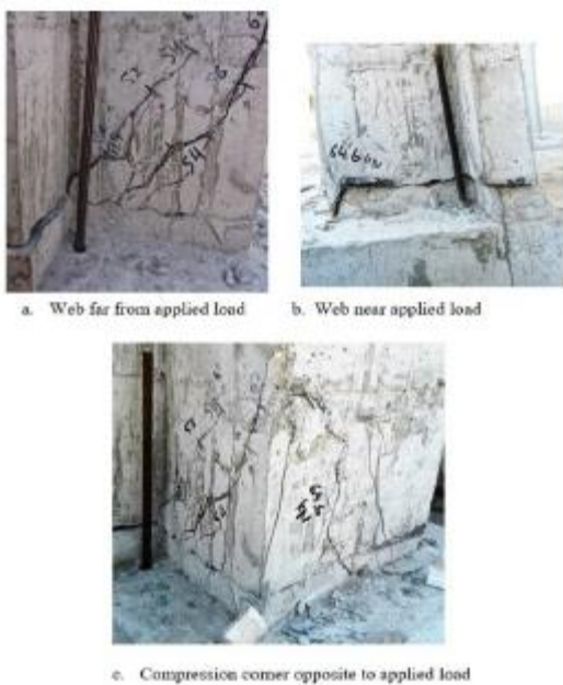
Fig. 13 Crack pattern of specimen (S3s-0.5Pys-0.4P)
