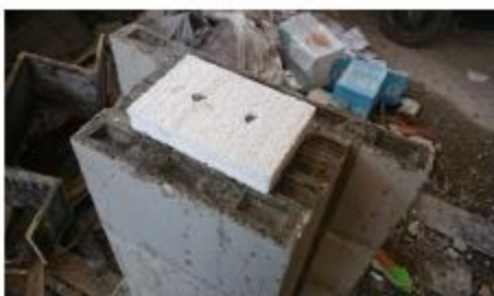
Fig. 6 formation of shear keys at joints
