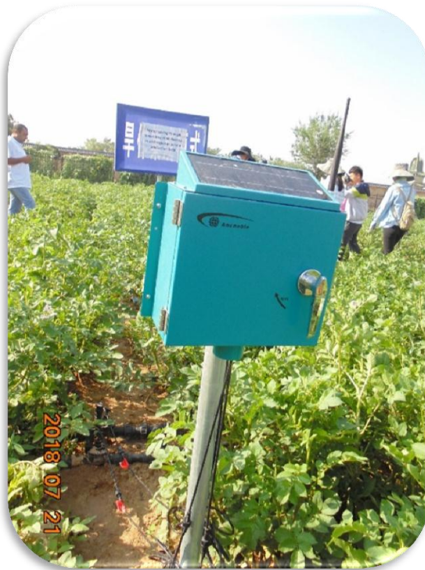
Irrigation controller unit with moisture sensor powered by solar energy
