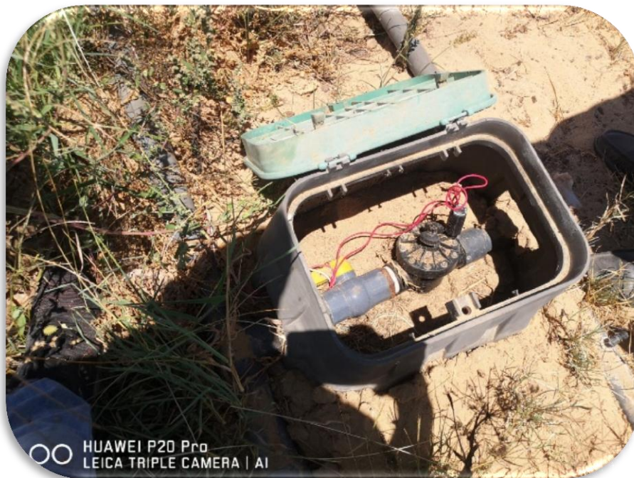
Solenoid valve used open and close irrigation water by timing of control board
