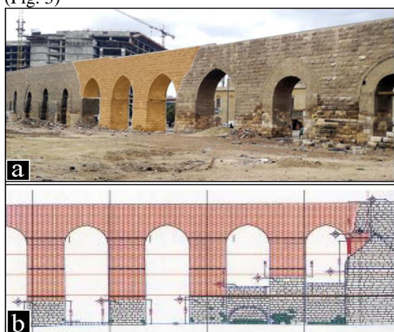
Fig. 3 a. The current condition of the Cairo citadel aqueduct, (b) sketch shows some newly completed arches
