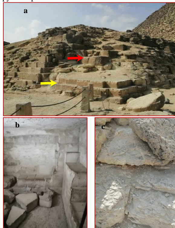
Fig. 2. (a) General view of Hetep Heres pyramid showing the main construction blocks "red arrow" and casing stones "yellow arrow", (b) the bed rock of the plateau, (c) detail of the rock-cut burial chamber.
