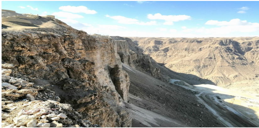
Fig. 7. Kinematic analysis of station 5. a) Plane failure potentiality. b) Wedge Failure Potentiality. Red points are critical intersections of joint planes daylighting slope. c) Toppling Failure Potentiality at S5.
