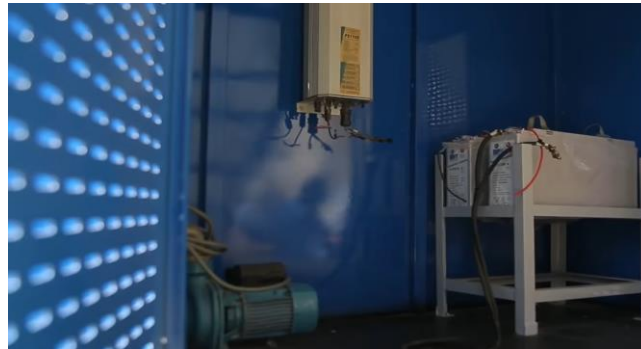
Fig. 4 Internal system components of the mobile solar water pumping system
