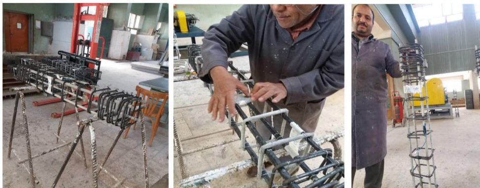
Fig. (6): preparing Cages of Column
