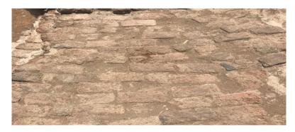
(Fig.11): Remains of the northern wall showing the construction method used to construct the basin.
