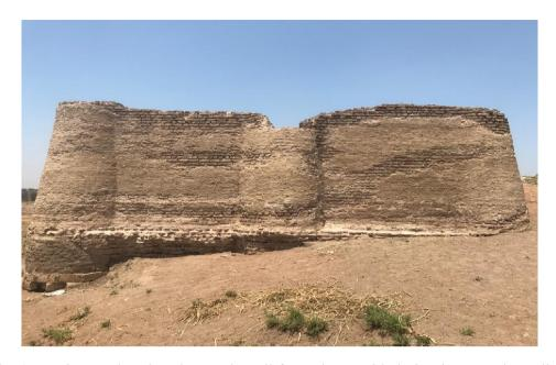
(Fig.6): A picture showing the south wall from the outside being in a good condition. (Photographed by the researchers)
