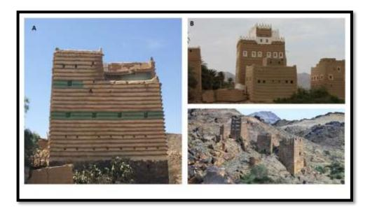
Fig.3. Models of heritage villages in Asir, (A) style mixed between stone and mud, (B) mud building style, and stone building style.
