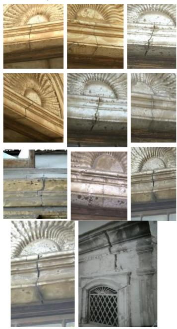
**Figs. 32 - 42** Display cracks of  $2^{nd}$  type in the springings of all lintels above openings in the mosque at positions of heavy load, the lower left photo. From Supreme Council of Antiquities archives (1935).
