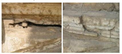
**Figs. 154- 155** Display the crumbling which is Detachment of larger, compact stone elements in the form of crumbs, in Egyptian alabaster of Muhammad Ali Mosque and not observed in chapels at Karnak.
