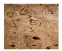
**Fig.73** display the vugs repair in the surfaces of the travertine of chapels at Karnak of Wadi El-Assiuty
