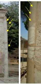
Figs. 43-47 Display frailty and debility structure of some ornamental architectural elements of Egyptian alabaster chapels at Karnak such as the Cavetto Cornices and torie which are along the horizontal upper edge and along the corners of the façade of them , in addition to being hanged partially on space, have exposed them to fracture and loss or to erosion (arrows).
