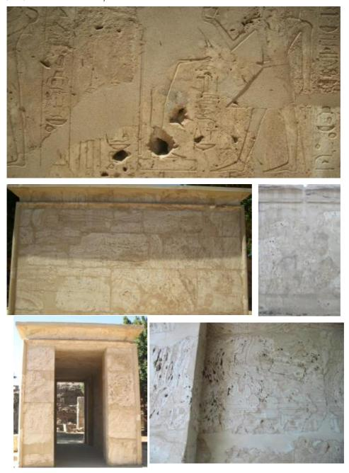
**Figs. 91- 95** Display the Bleaching of the exterior surfaces of the chapel of Thutmosis IV at Karnak and other adjacent alabasterite chapels Where the coloring of honey , pale-orange , pale yellow , brown or pale tan to yellowish white with an orange tint are bleached or faded to white color due to exposure to the sun .
