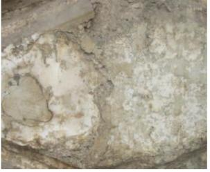
Fig.156 Display flaking to contour scaling, in Egyptian alabaster of Muhammad Ali Mosque and not observed in chapels at Karnak.
