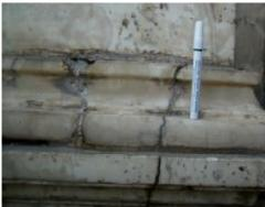
**Figs. 28-31** the first type of cracks which are usually short and isolated involving small deformation of masonry , and they are distributed randomly and irregularly over the whole building - is related to both the physical and chemical properties of materials and constructional methods
