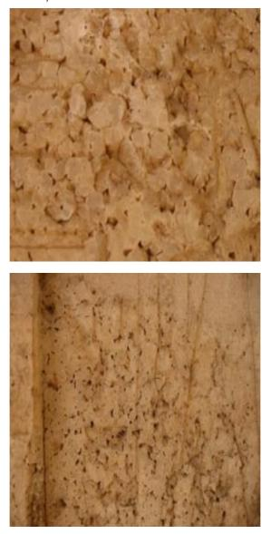
**Figs. 74-75** Display superficial coarsening and granulation on the surfaces of the travertine of chapels at Karnak smoothed by corrosion polishing as external deterioration factors.
