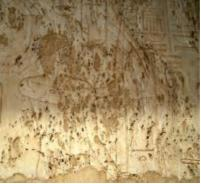
**Figs 65-66** display the first type of vugs and open spaces is a minute cavities of distribution throughout the surfaces of the travertine of chapels at Karnak of Wadi El-Assiuty, and they were stained with red ironoxide
