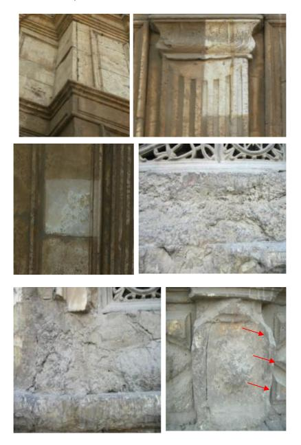
**Figs. 102-107** Muhammad Ali Mosque show that the soiling areas easily removed and another type of soiling is not easily removed, also here there is a thick black crusts of irregular shape or discoloration (soiling) to crust are just an extreme case of the lower right photo, Since such crusts are brittle and tend to detach from the alabaster (red arrows).
