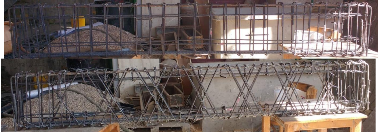
Fig.18-b. Reinforcing steel cage for solid and castellated beams.
