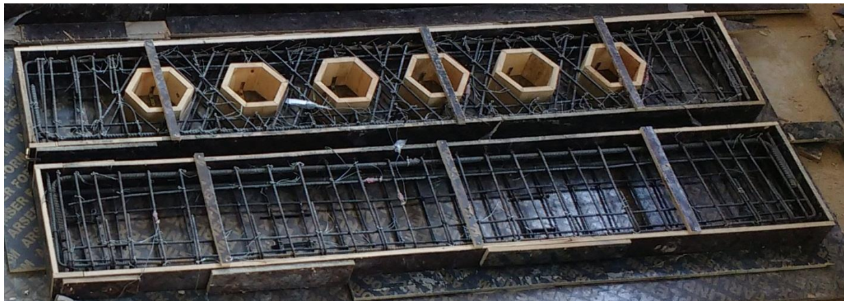
Fig.18-c. Solid and castellated beams just before casting.
