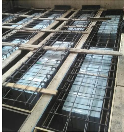
Fig. 2 Image showing steel cages just before casting of the test beams.
