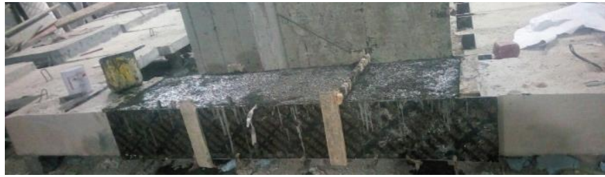
Fig.6 Image showing the ECC pouring for beam B-ECC.
