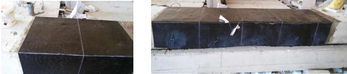
Fig. 4 Images showing CFRP sheets after application on beam B-CFRP.
