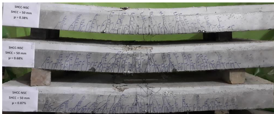
Fig. 8 Final crack pattern of specimens of group (II).
