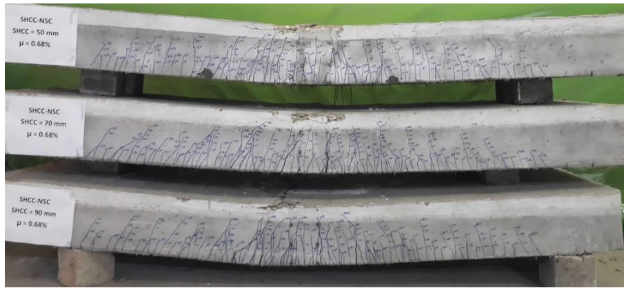
Fig. 9 Final crack pattern of specimens of group (III).
