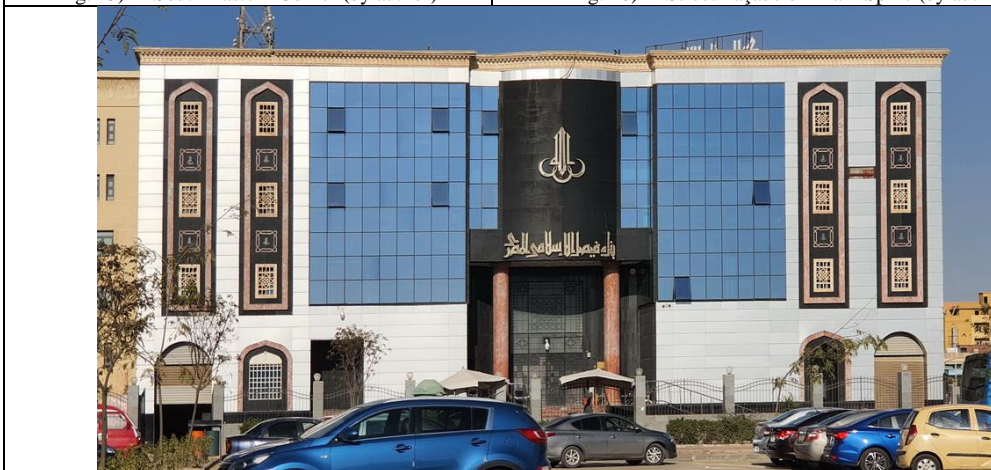
Fig. 17) Main Entrance Façade (by author)
