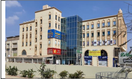
Fig. 19) Southern façade (by author)
