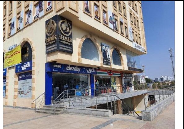
Fig. 22) Detail of the lower segment of Main Façade. (by author)
