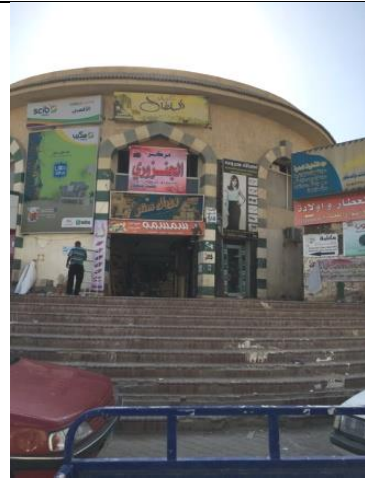
Fig. 4) Entrance from the North West Corner (by author)
