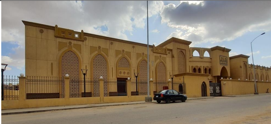
Fig. 37) Street Façade, Eastern Segment (by author)
