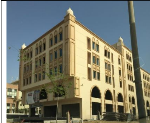
Fig. 21) Main Street Façade (by author)
