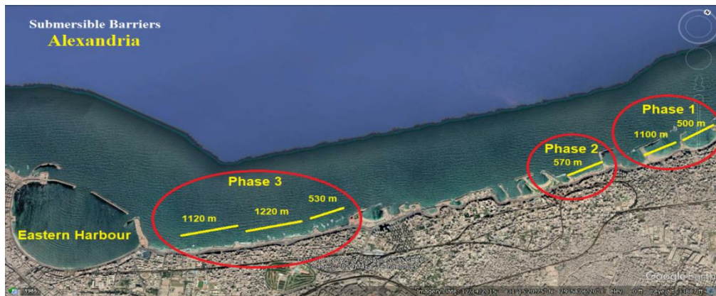
Figure .7 Submersible Barriers Project in Alexandria
