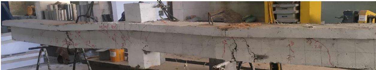
Fig. 6. Failure mode of beam BS3.
