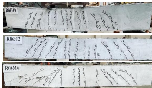
Fig. 8: Crack pattern of specimens in Group 2 at failure
