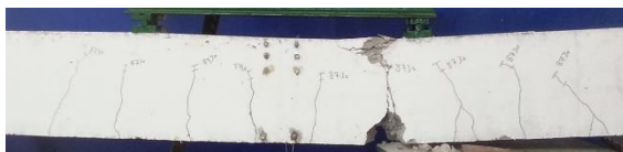
Fig. 8: failure mode of beam BC
