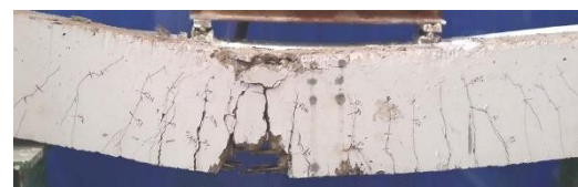
Fig. 11: failure mode of BF
