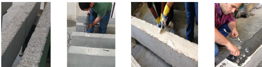
Fig. 4 E.B. steel plate with end anchors application process
