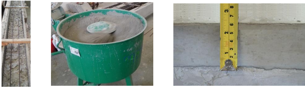
Fig. 5: Applying UHP-SHCC layer process
