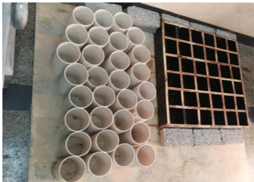
(b) Preparing the forms
