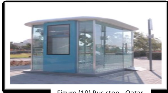
Figure (19) Bus stop - Qatar
