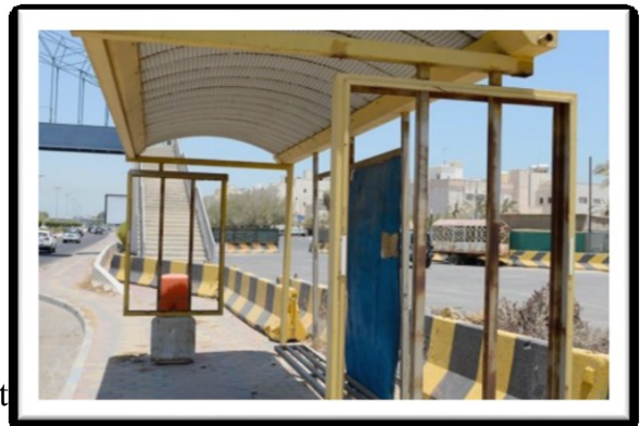
Figure (10) Two traditional Bus Stop Shelter - Kuwait
