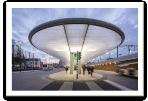
Figure (2) Casar De Caceres Bus Station -
