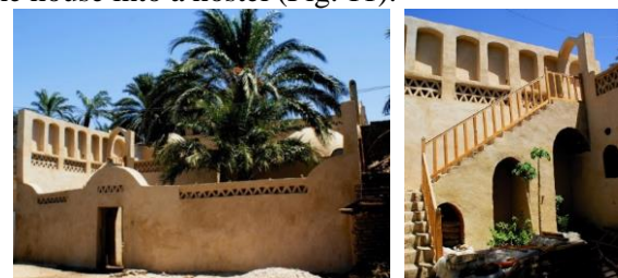
Figure. 11 The conservation initiative carried out on one of the houses designed by Hassan Fathy in
