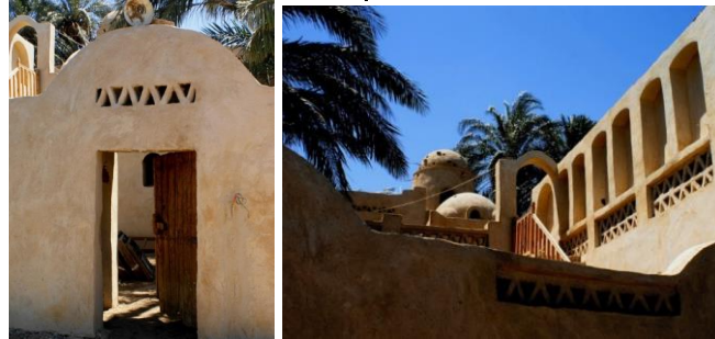
Figure . 12 The gate of the house designed by Hassan Fathy in New Gournia, which was the subject of the conservation and rehabilitation works ,b) The new dome and dovecot added to the house during the conservation works.
