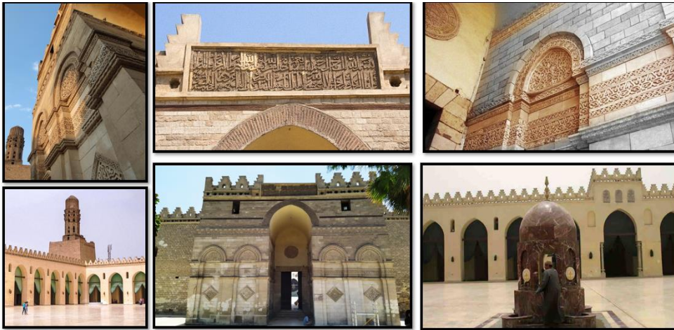
Fig. (6) illustrates the Architectural aesthetic values inside and outside al-Hakim bi-Amr Allah Mosque
