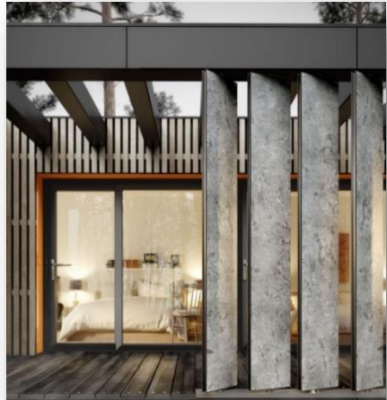
Figure (4) Shows Modern metal façade as new material used as sunscreen (pin.it.2022)
