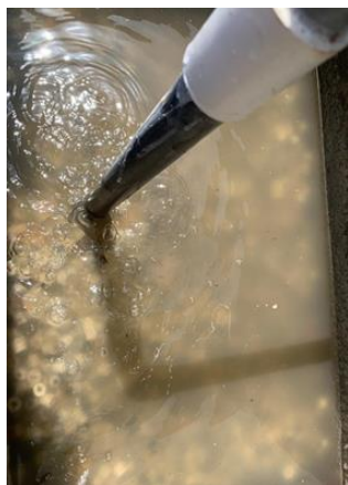
Fig (2) : The submerged ceramic ring media in the submerged aerated filter.
