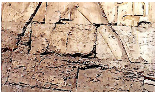
Fig. 46 displays the laminated or bedding limestone (Thebes and transitional Drunka formations ) in the adjacent calcareous lower Eocene plateau similar to in Seti I and Ramesses II temples at Abvdos
