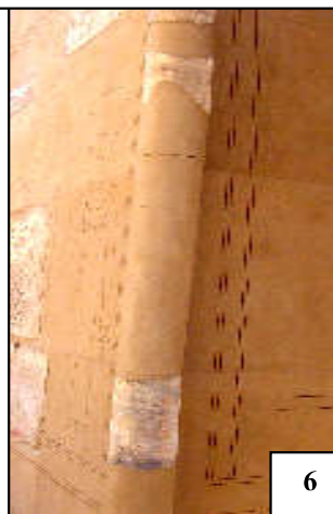
Figs.64 - 65) display the compensation with plastic repair (mortars) for the cavetto cornices , torie of the terrace of the second court and edges of staircases and balustrades of the staircases leading from the first to the second court of the temple of Seti I (64) and Ramesses II (65) at where the plastic repair is more suitable for formation and reconstruction of many of the ornamental and architectural elements with accuracy and homogeneity plus the possibility of addition of chemical additives to mortars to increase resistance of friction of the infantry, also prevents from disturbing fragile areas .
