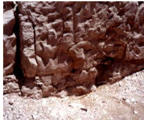
Fig. 45 displays Oolitic texture in the inside southern wall at the temple Ramesses II at Abydos similar to in the adjacent calcareous lower Eocene plateau
