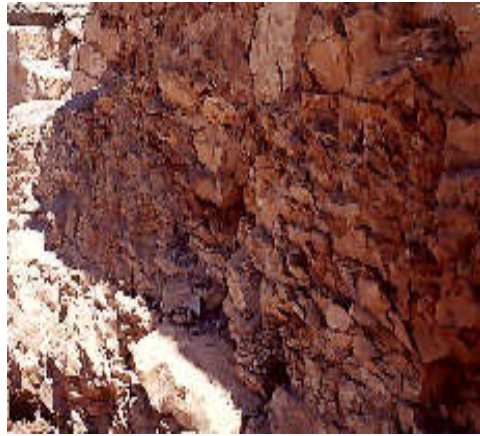
Fig. 43 displays Oolitic structure in remains of the north tower of the first pylon of Seti I temple at Abydos similar to in the adjacent calcareous lower Eocene plateau
