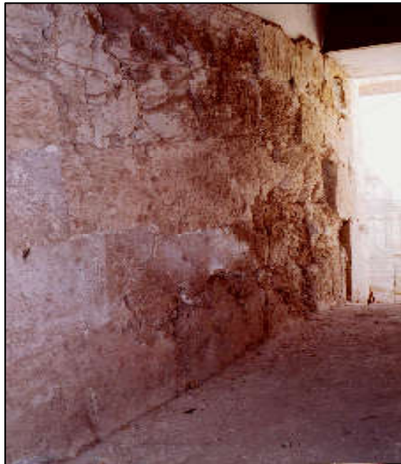
Fig.4 Display an example of loss and absence of archaeological stone building structural, functional and esthetical role in addition to loss of inscriptions , drawings and paintings (documentary and esthetical function ) in the funeral passage Osireion at Abydos because of raising of ground water tables and continuous salt crystallizing , so we have to remove deterioration and damage causes and sources before replacement with original local limestone
