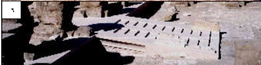
Figs.64 - 65) display the compensation with plastic repair (mortars) for the cavetto cornices , torie of the terrace of the second court and edges of staircases and balustrades of the staircases leading from the first to the second court of the temple of Seti I (64) and Ramesses II (65) at where the plastic repair is more suitable for formation and reconstruction of many of the ornamental and architectural elements with accuracy and homogeneity plus the possibility of addition of chemical additives to mortars to increase resistance of friction of the infantry, also prevents from disturbing fragile areas .
