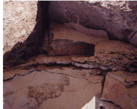
Fig. 47 displays the laminated or bedding limestone (Thebes and transitional Drunka formations ) in western wall of Ramesses II temple at Abydos similar to in the adjacent calcareous lower Eocene plateau .
