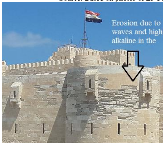
Fig (6): Erosion in walls due to high alkaline in the air and waves action.
