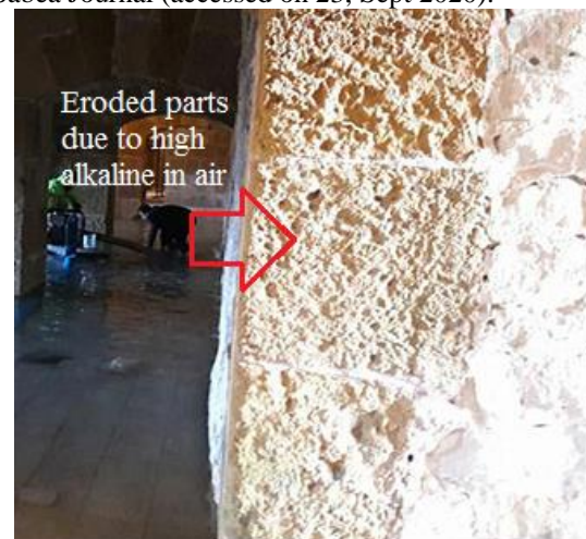
Fig (6): Erosion in walls due to high alkaline in the air and waves action.
